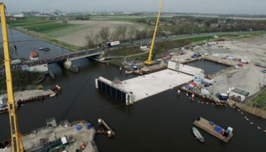
Work on the N31 road is taking place in Harlingen. In the future, the new road will cross the canal with an aqueduct. This aqueduct was transported by boat to its final location in the canal in the spring of 2017. Other activities will produce little to no hindrance for the shipping traffic. At the end of the year, the Koning bridge (Koningsbrug) at Harlingen will be renovated. This may cause some hindrance.
